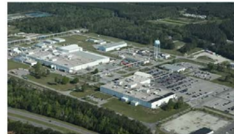
GE Vernova plant in Eunice, New Mexico. (Image: GE Vernova)
